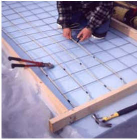
Floorizwarm Heating Element Layout
